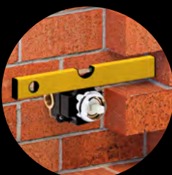
Leveling of the concealed part.
