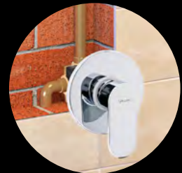
Installation of external components.
